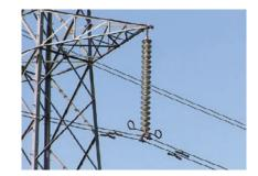
Insulators are useful for separating electricity from objects and living things that it could damage. In the picture at the left, power lines are separated from the metal tower by a stack of ceramic insulators.
