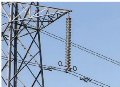
Insulators are useful for separating electricity from objects and living things that it could damage. In the picture at the left, power lines are separated from the metal tower by a stack of ceramic insulators.
